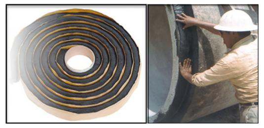
These Cold Adhesive Preformed Plastic Gaskets are generally not seen used currently on reinforced concrete pipe.
